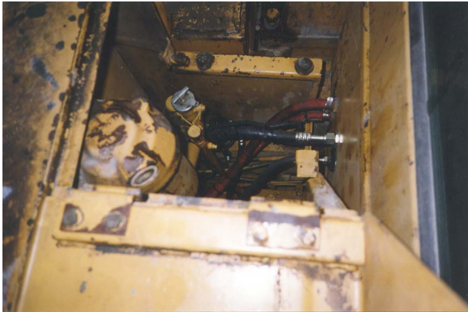
Drier in place with hoses.
